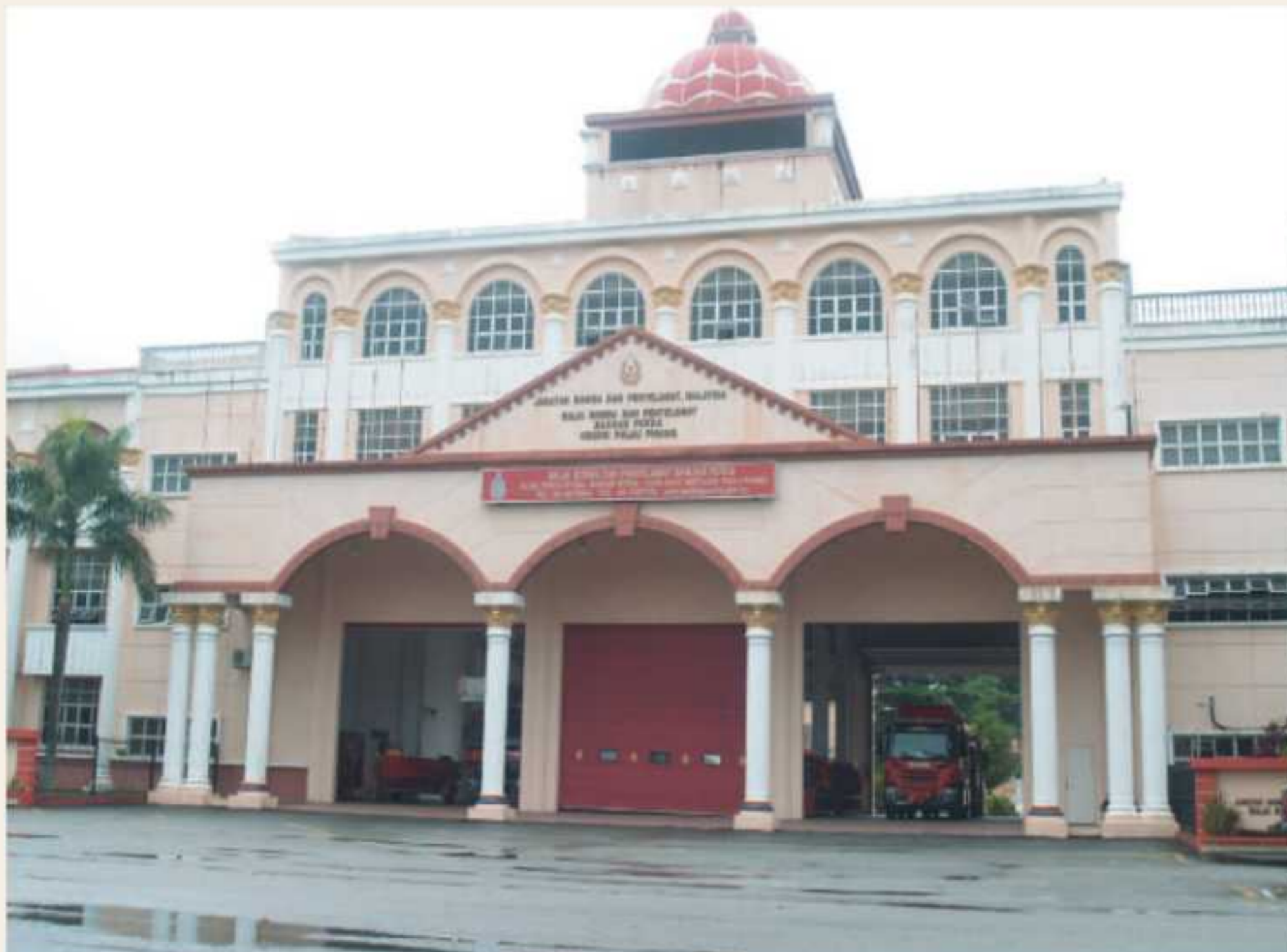
Malaysia Fire and Rescue Station, Perda, Pulau Pinang
